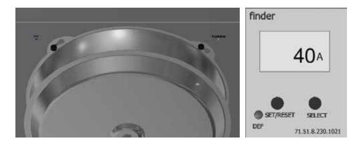
Take down a grease collector in the kitchen hood closest to Jeven UV-Control, read which current value is now displayed on the Finder 71.51 when a UV-lamp has been turned off.
