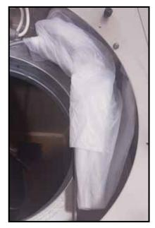
8 Encapsulate luminaire and light source with tight plastic bag
